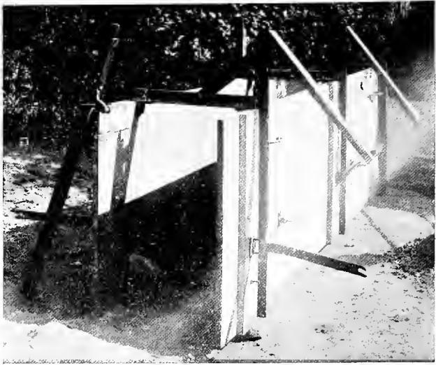
MARK V SHUTTERING.
